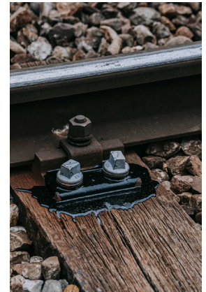
Figure 2: SLS Installed in Old Ties
