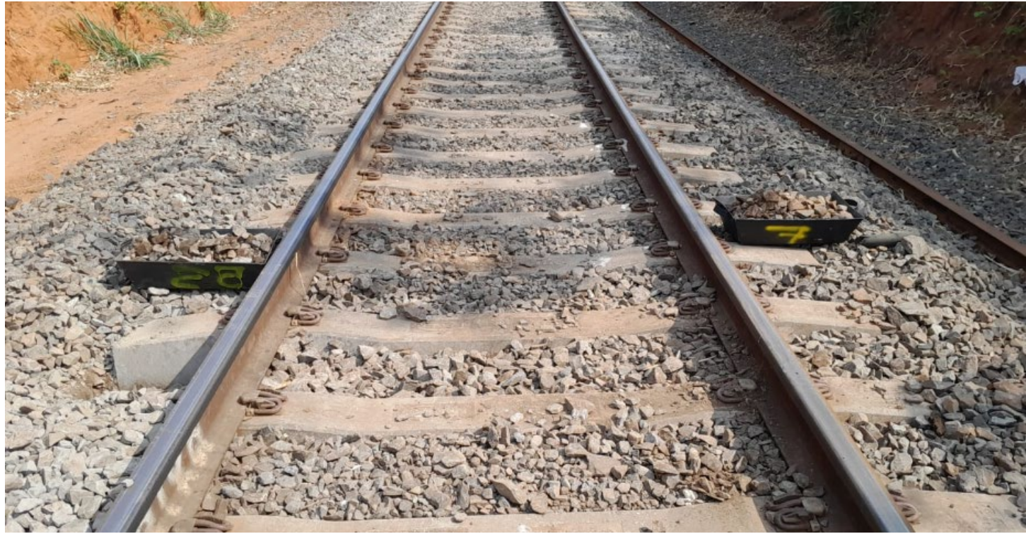
Figure 2. Example of ballast sample collection
